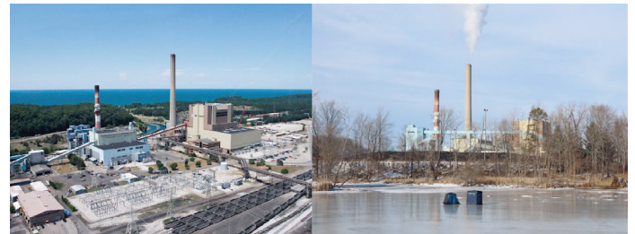
The Consumers Energy J. H. Campbell Coal Plant
